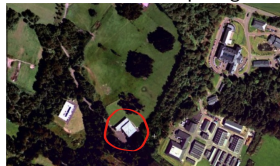
EPCC Advanced Computing Facility, 2014
